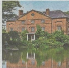
Bossington Mill on the River Test in Houghton, Hampshire, is on sale for £2.4 million with Strutt & Parker
